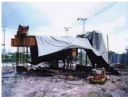
Static Axial Pile Load Test
