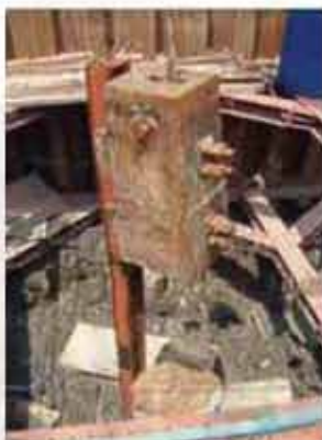
Dynamic Axial Pile Load Test
